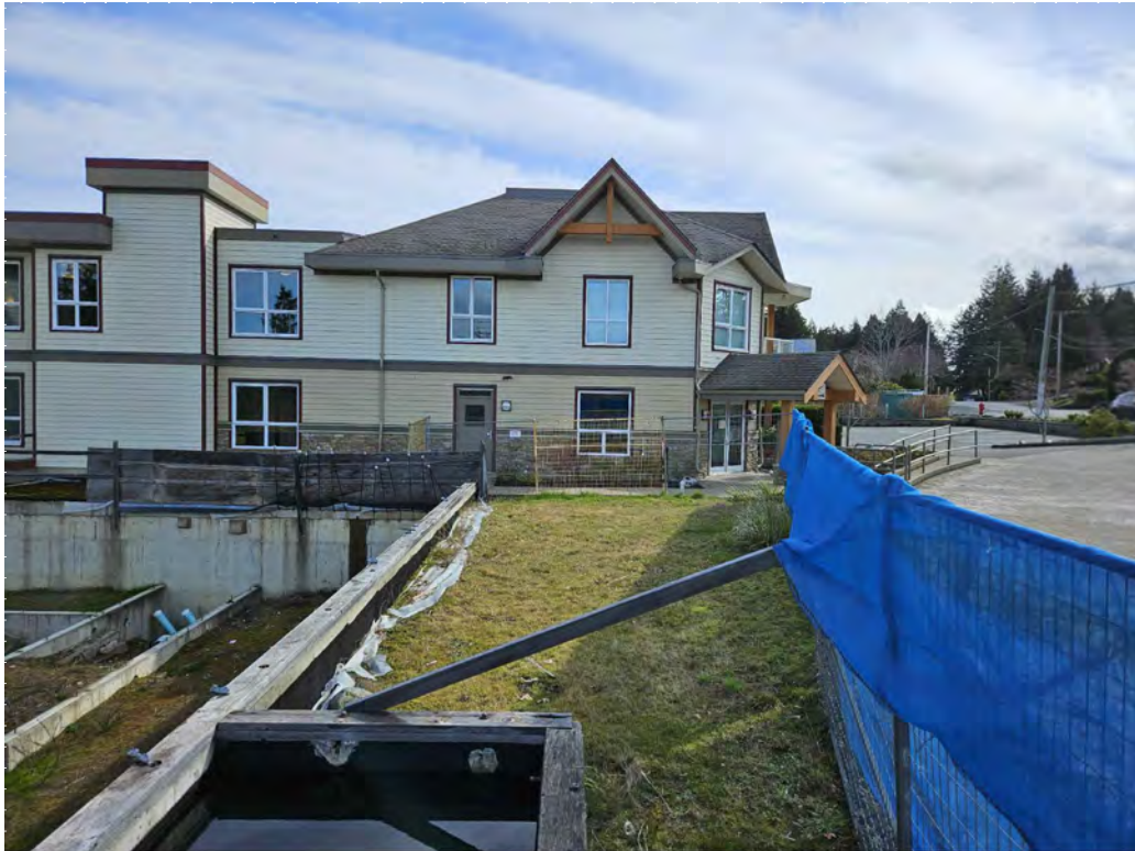
BUILDING AT EAST SIDE
