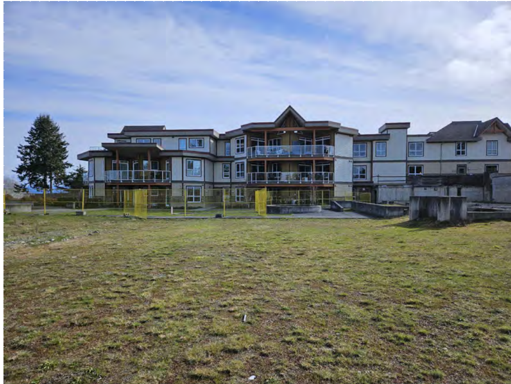
BUILDING AT EAST SIDE
