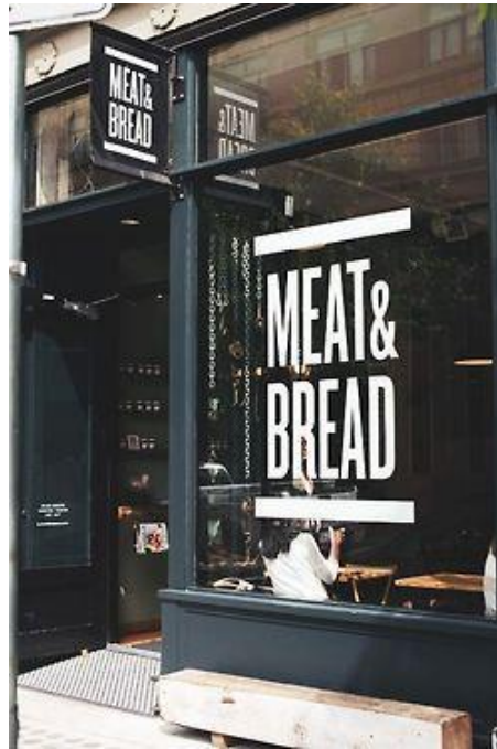
Traditional open storefront designs with bulwarks, display and clerestory windows, and recessed entries are recommended.
