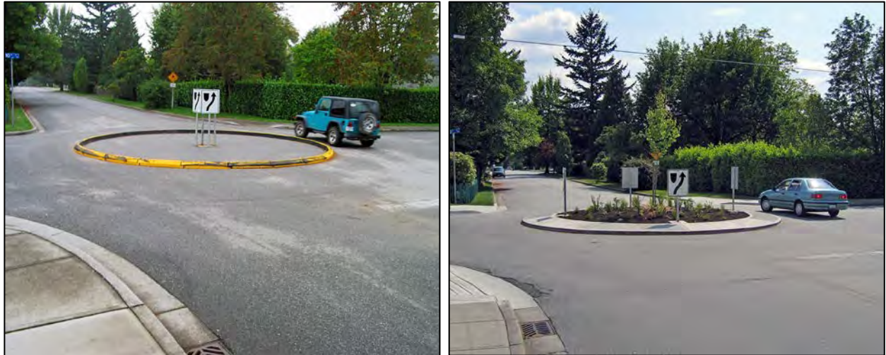
Figure 2.9: Temporary and permanent traffic circles
