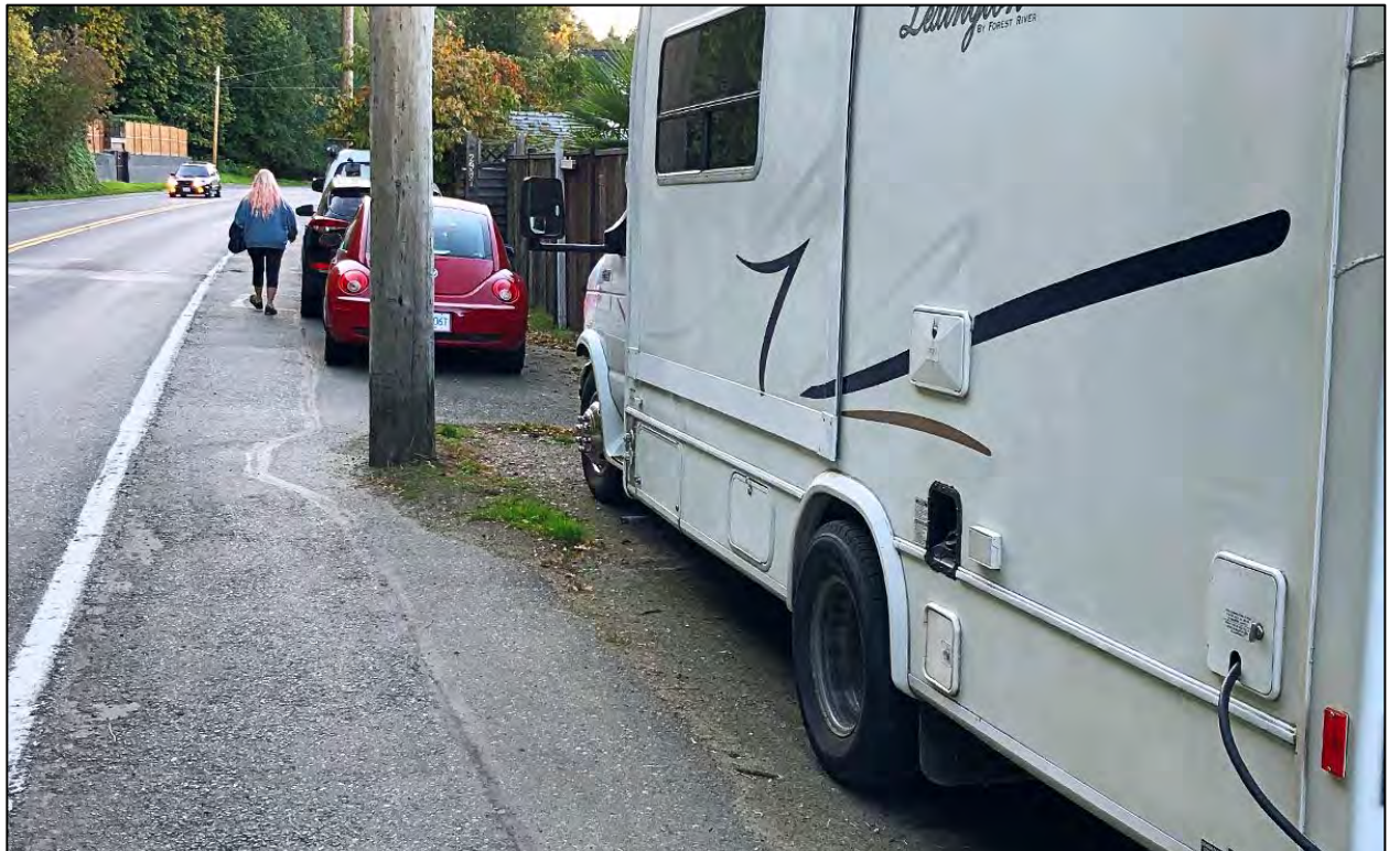
Figure 2.7: Prohibit parking on shoulder less than 4 m wide, Highway 19A
