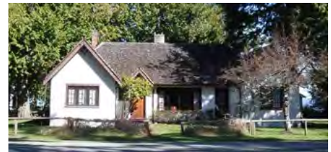
The existing lodge building is an aging structure and will require upgrading or replacement in the near future
