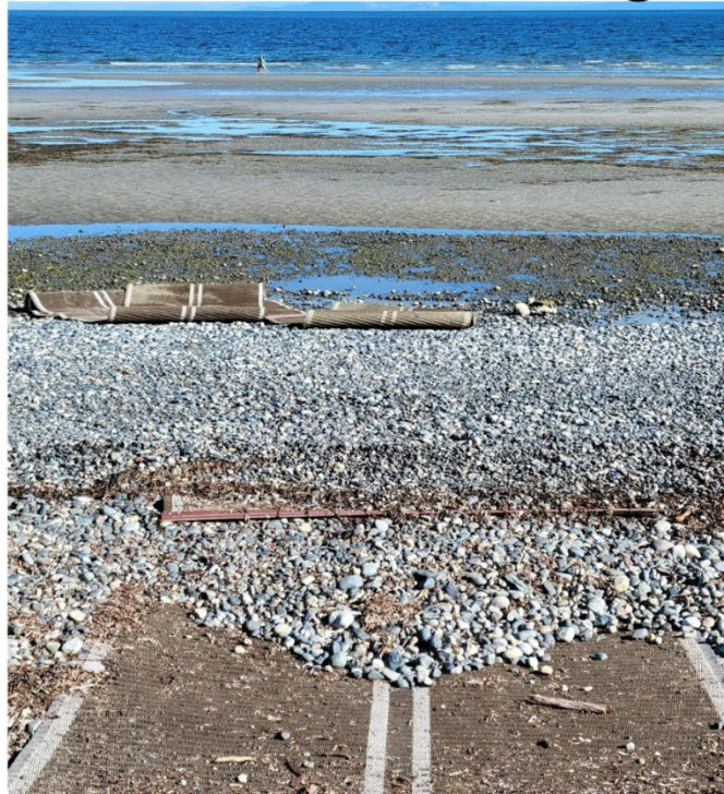
Torn mat and covered in gravels
