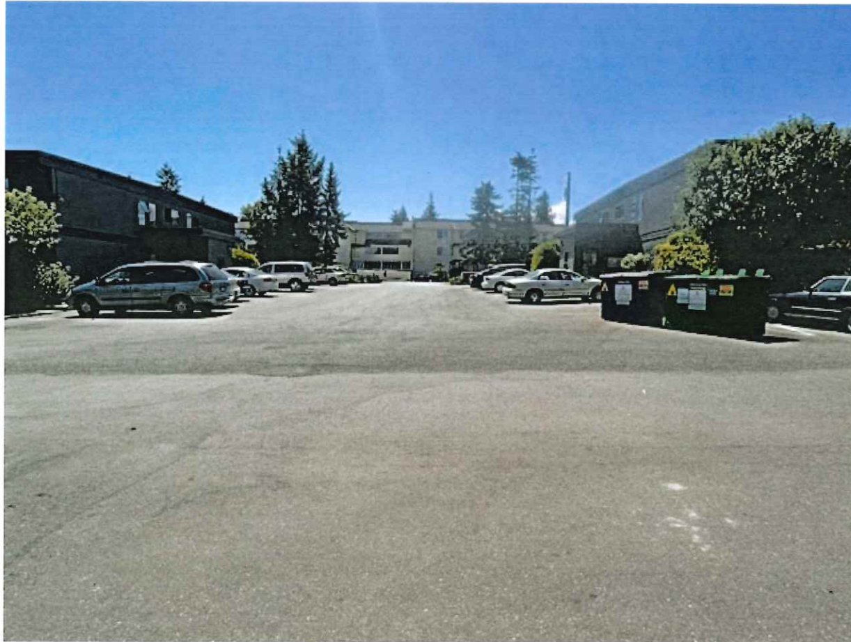
Looking South Between Buildings From Back Lane
