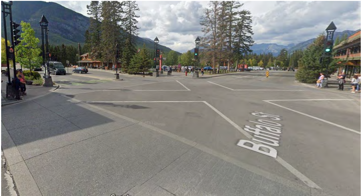
Figure 5.1: Paint Markings at an Intersection with Pedestrian Scramble Signal Phase
