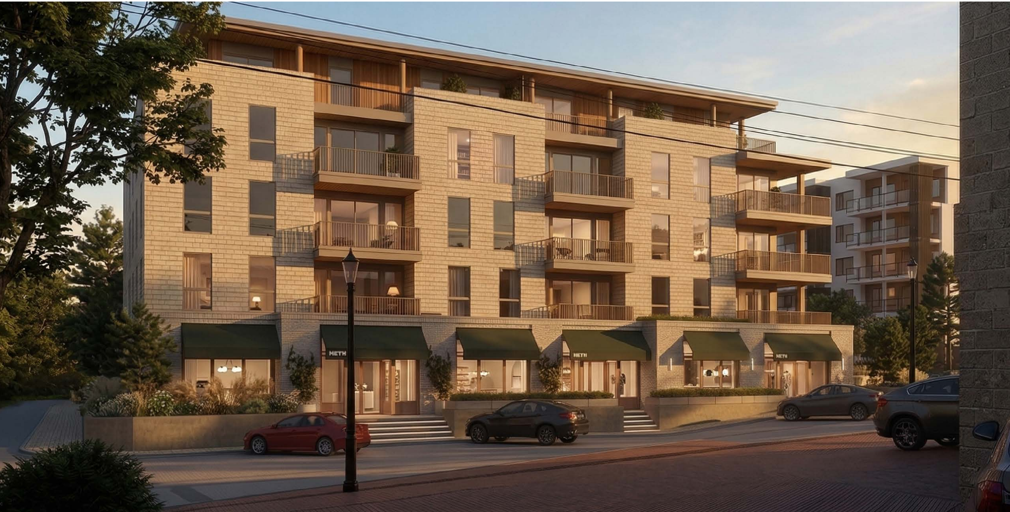
WEST ELEVATION FROM HARLECH RD
