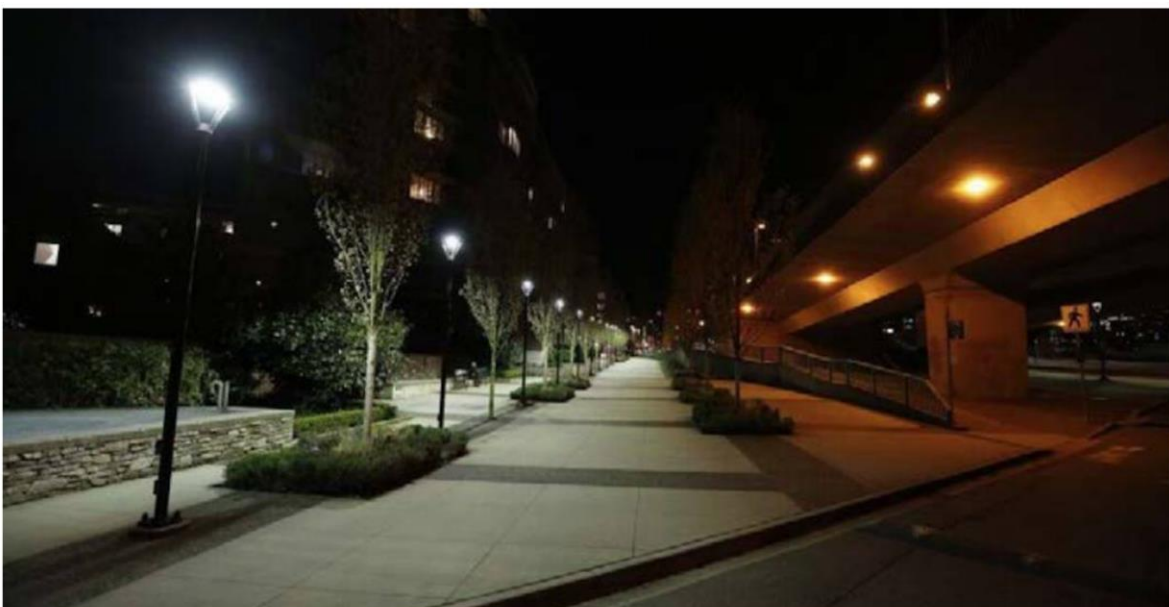
LED lights on a pedestrian pathway (left) and HPS lights (right) at the south end of the Cambie Street Bridge. (City of Vancouver)
