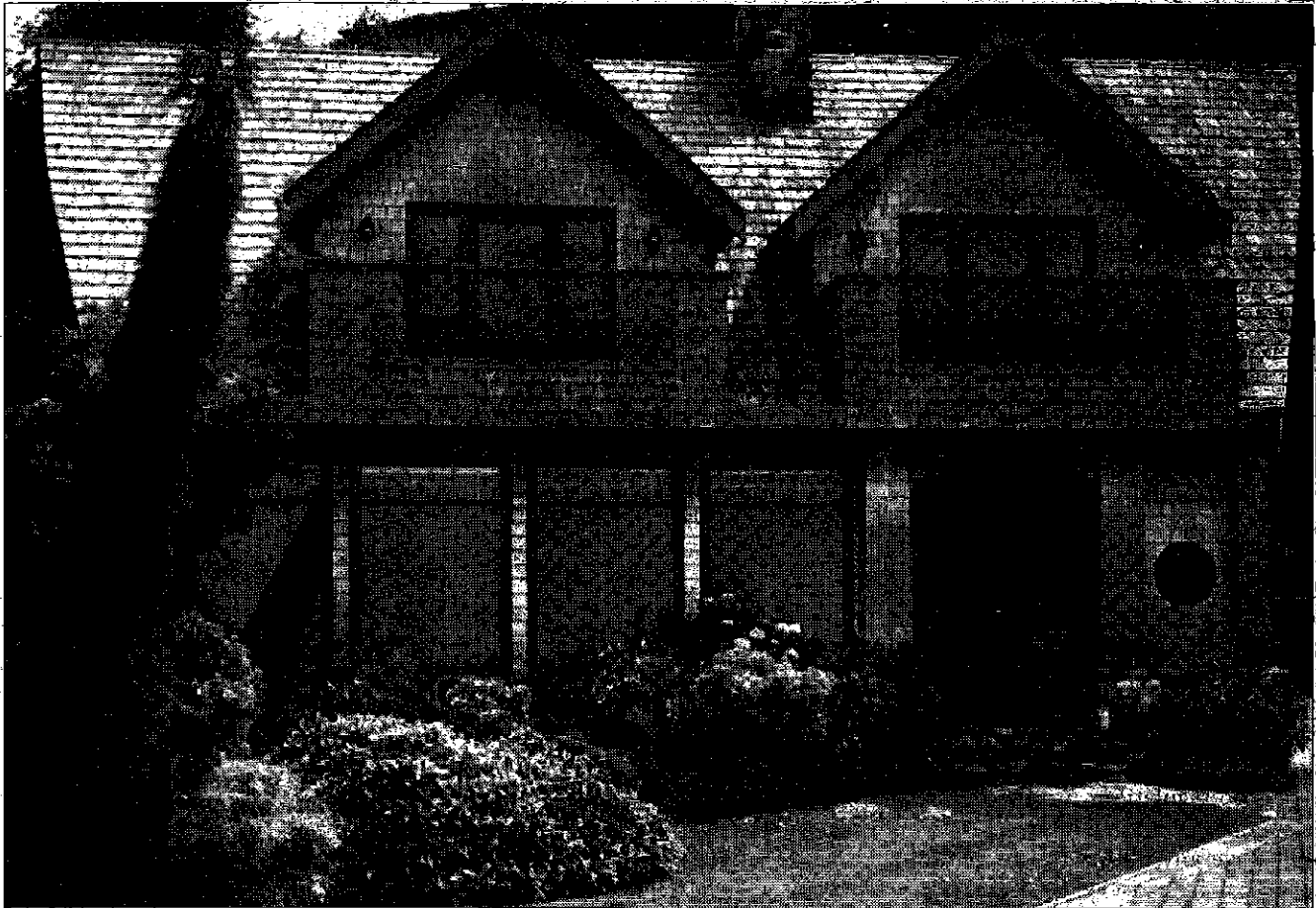
Homes like these will be on display, in an effort to raise funds to purchase the remaining Brown property.
